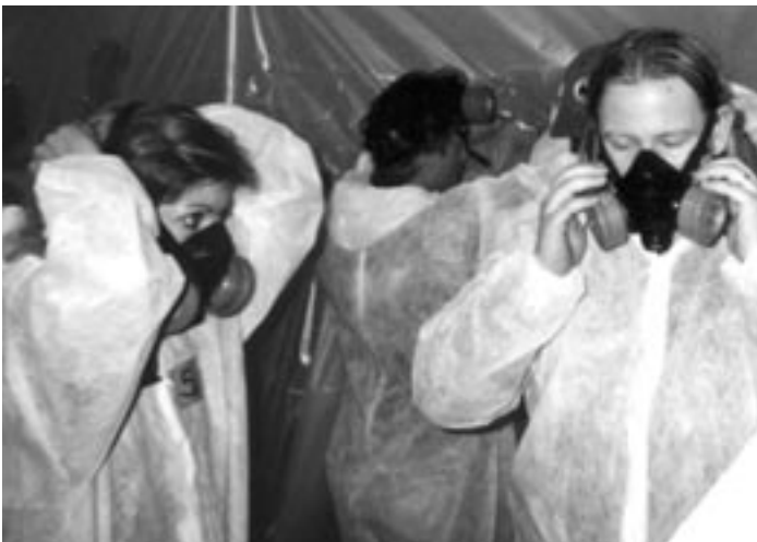
SKOOKUM ABATEMENT SERVICES: Employees don protective gear before entering a contaminated area.
